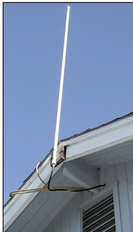
Figure 5—The completed antenna mounted to the roof.
